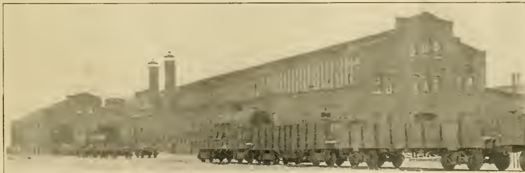
VIEW OF FOUNDRY FROM NORTHWEST CORNER, SHOWING CUPOLAS AND STOCKHOUSE AT LEFT.
